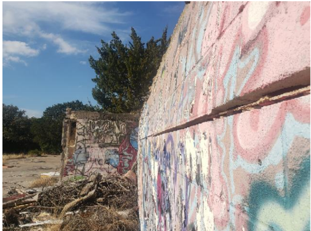
Figure 03. Faulting of upper wall
