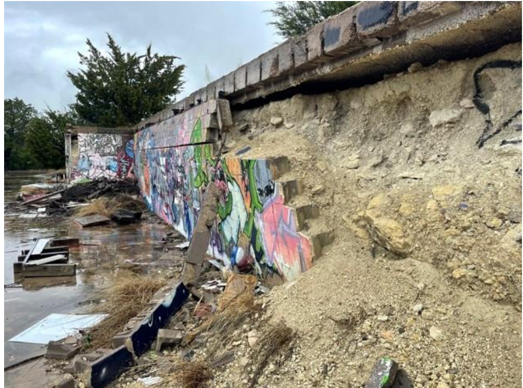
Figure 02. Partial collapse and buckling of upper wall
