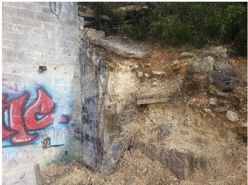
Figure 07. Partial collapse of wall return at east side of lower wall
