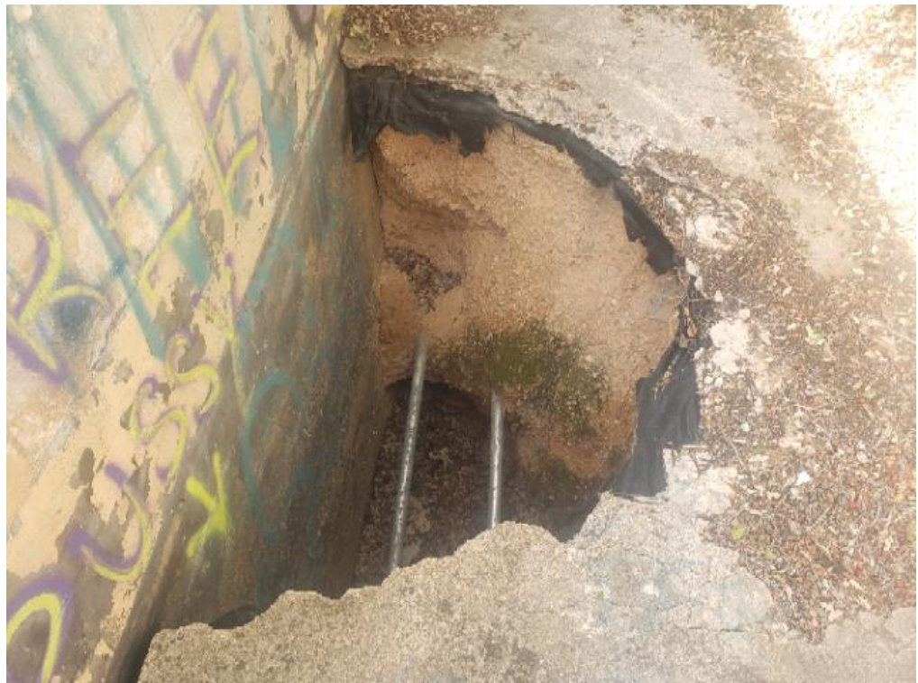
Figure 08. Holes in flatwork behind lower wall, due to soil cave-in
