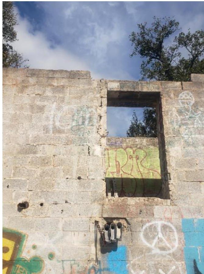
Figure 09. Cracking in jamb blocks supporting lintel, lower wall
